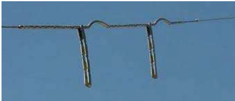
Fig. 7- Anti-twisting Devices
