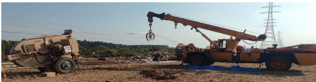
Stringing Setup Equipment Alignment
