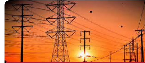
Power Transmission & Distribution
